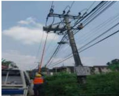
Gambar 7. Proses Pelepasan *Disconnection Switch* (DS)
