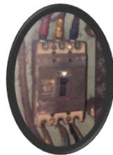
Gambar 6. Molded Case Circuit Breaker (Dokumen Pribadi)
