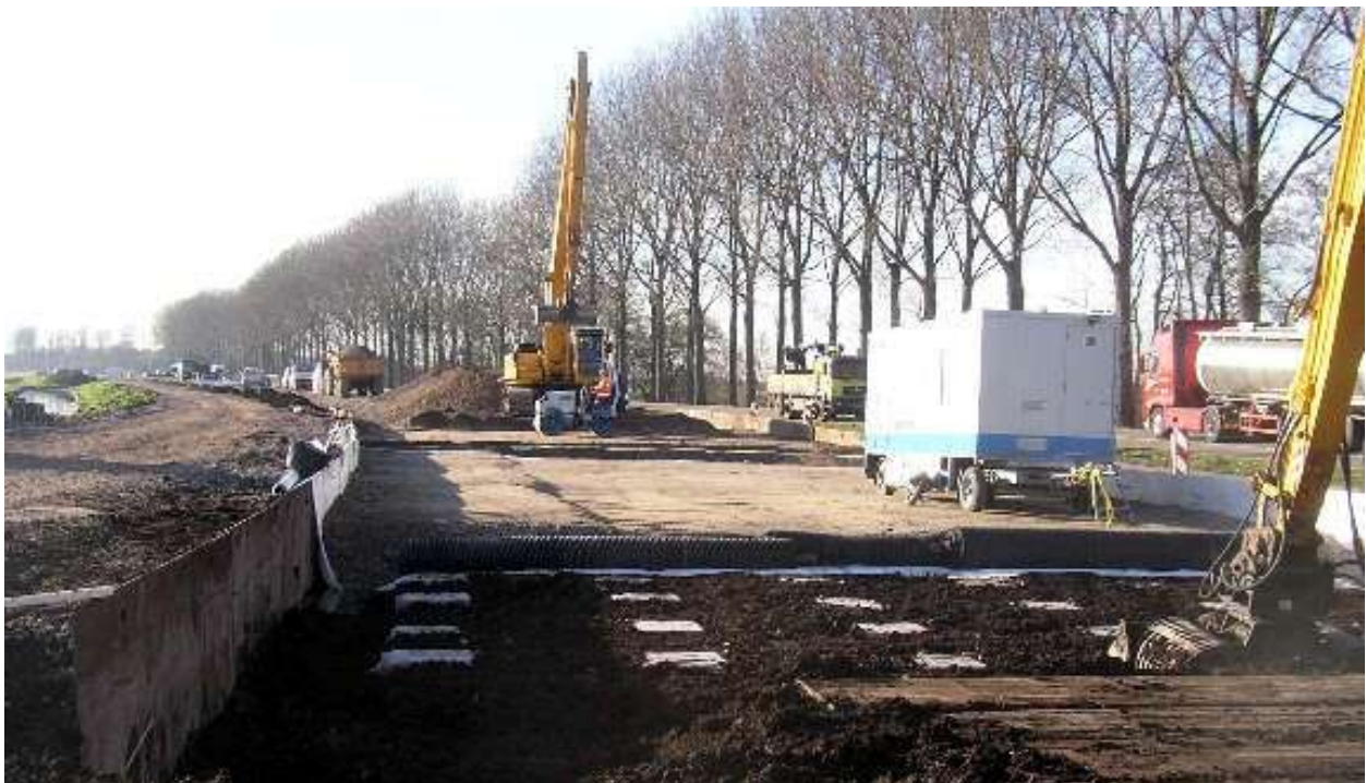
Figure 1. Implementation of pile embankments (Esseveld, 2024)
