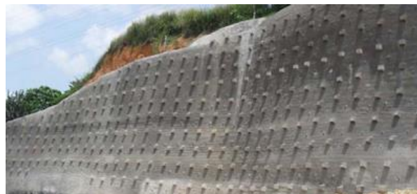
Gambar 2. Dinding penahan tanah tipe soil nailing (Hardiyatmo,2006)
