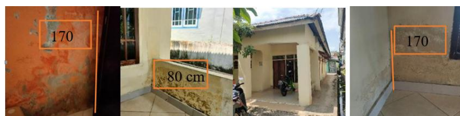
Figure 3. Flood marks are visible on the house's walls. Source: Authors, 2023
