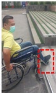
Figure 9. The ramp is less sloping, thus hindering the movement of wheelchairs Source: personal documentation, 2022
