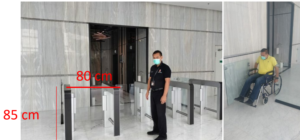
Figure 14. A special door for wheelchair users at the entrance to the lobby office Source: personal documentation, 2022
