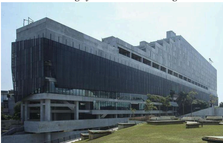
Revitalized Building of The DKI Jakarta Regional Public Library in Cikini
