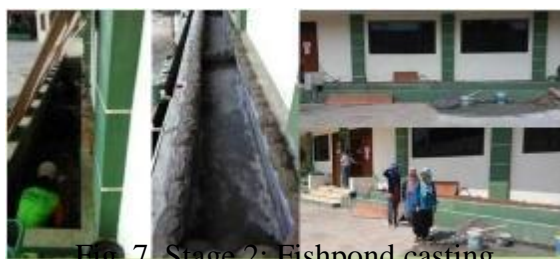
Fig. 7. Stage 2: Fishpond casting (Source: Team's Documentation, 2017)
